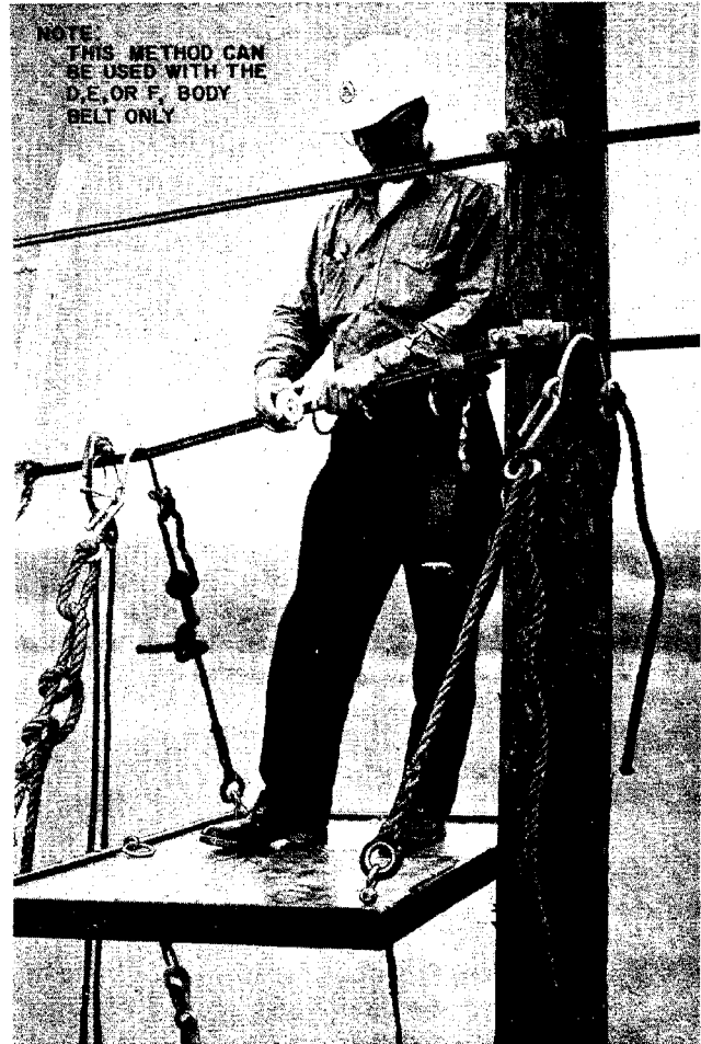
Fig. 9—Method of Using D, E, or F Body Belt With Safety Strap on Self-Supporting Cable
